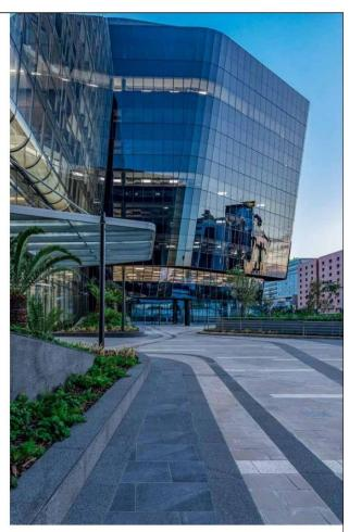
and baked with a variety of chemicals to reflect heat, so while it allows natural light to enter, heat wavelengths are reflected back out of the building. There was no laydown area available on the site, so all facades were prefabricated off-site then installed immediately on delivery, which had to be tightly planned and co-ordinated.
