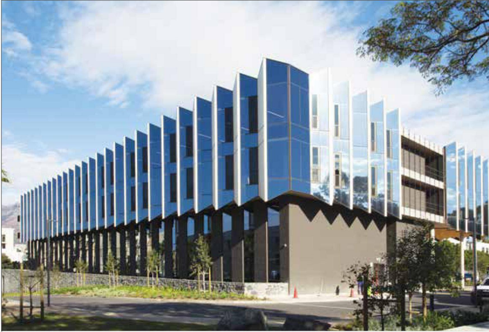
The function of the sawtooth CLT façade corrects the north-south line, meaning that the sun in the east strikes the CLT panel and can't directly enter the building.
