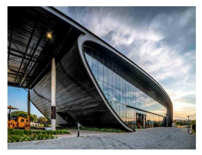
A steel girder framework provided the tracked-shape design of each of the two bubbles, with large spanning trusses carrying the roof, all sitting on a speciallydevised grid to accommodate the different sized equipment required. The two ends of the building consist of curved structural steel and horizontal sheeting that both cantilever 15 m out from the base and are 15 m high.
