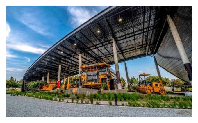
While the shape provided the volume and extent that such a showroom required, it also posed a range of structural challenges. The integrity of the 'bubble' design was ensured by maximising the grid distance and using steel as the main structural element.
