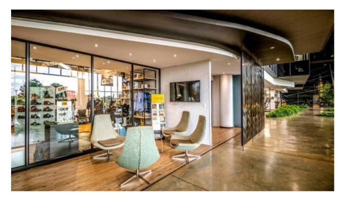
The flush-glazed unitised façade with performance-glass affords the main view into the showroom. An important benefit of the 'bubble' shape is that the canopy of the top edge has a 3.5 m cantilever, which not only gives excellent shading in summer, but is exposed in winter, which heats the internal space naturally.
