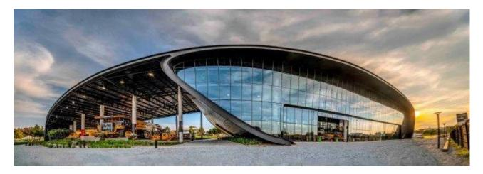
The 3 200 m2 showroom 'bubble' was built to face directly onto the R24, commanding immediate attention with its striking. It consists of two sections, one for tracked Caterpillar heavy industrial equipment and the other for machines with tyres. Architecturally the only straight feature in the double structure is the glass frontage. The curved roofs and sides had to seal with the straight lines to make the structures weatherproof and thermally-insulated.
