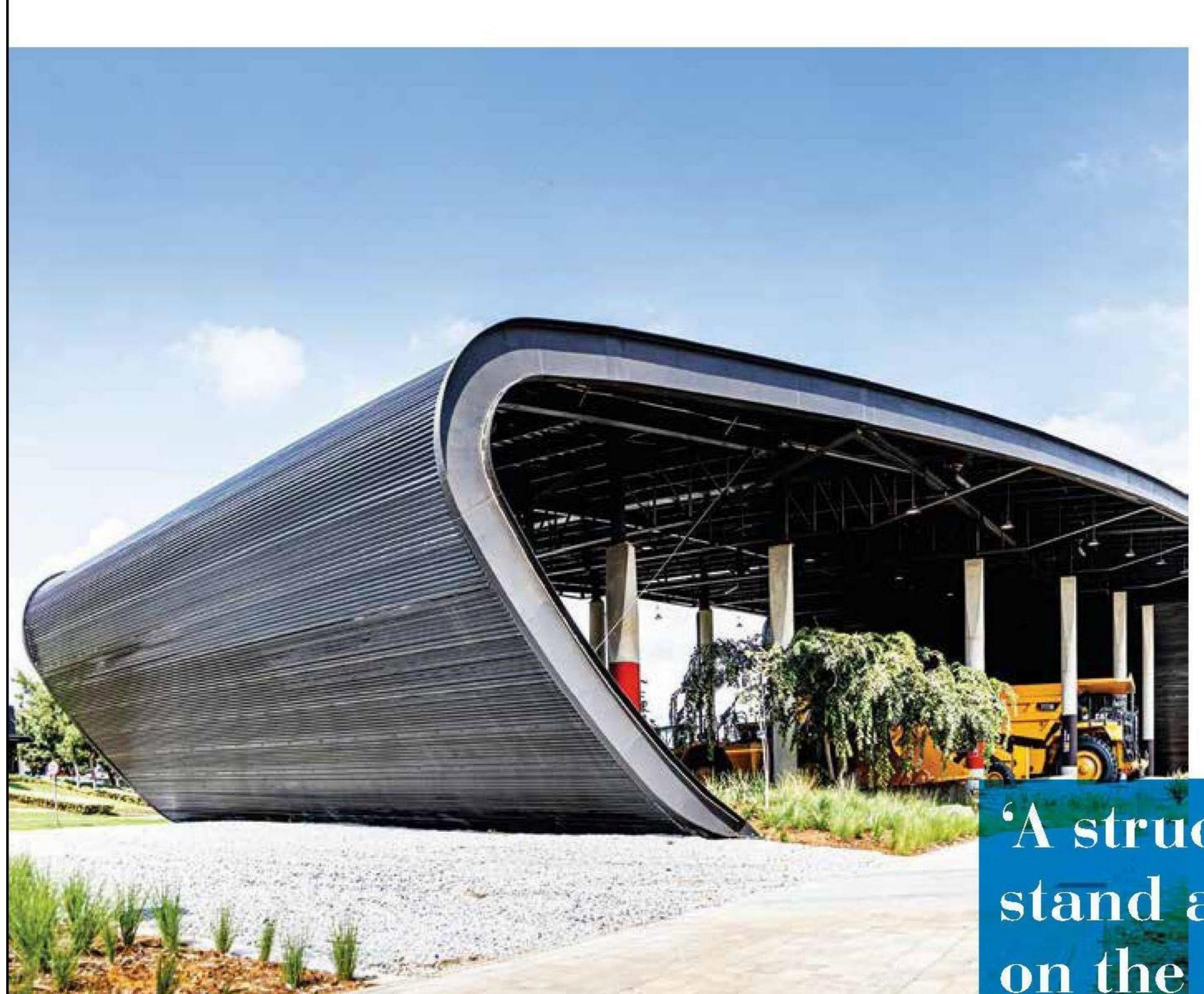
contracts manager Ernst Bezuidenhout. The steel structure was difficult to manufacture and erect, and they used tension cables in the roof structure to help with the installation of the glass and to adjust the fit of the facade panels.
