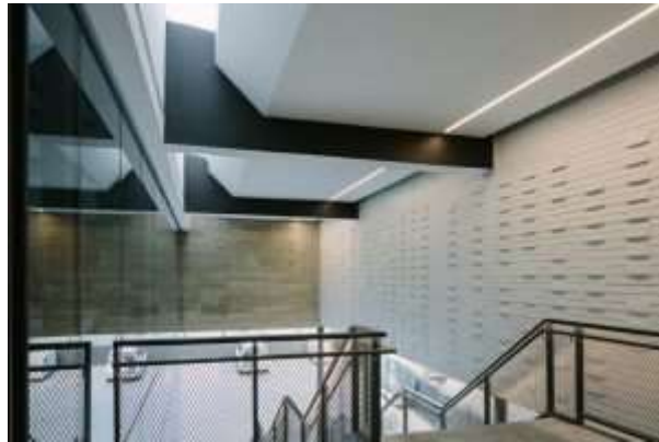
Pic: Opaque Poly-carbonate Skylights let natural light into the foyer
