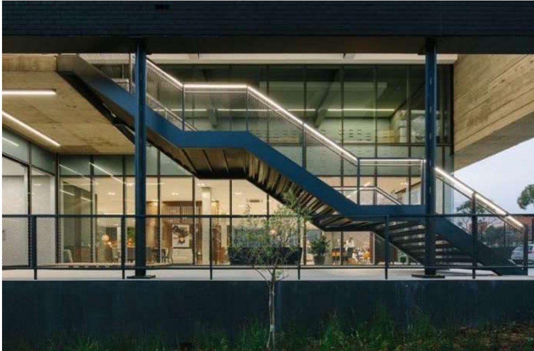
Pic: The open air foyer with industrial stair case featuring LED handrails
