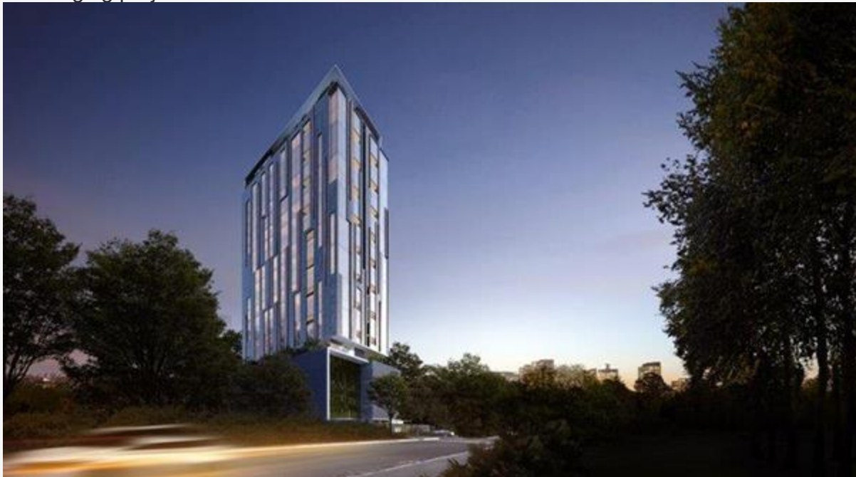
The 23-storey Habitat in Nairobi is Paragon's tallest building in construction to date.
